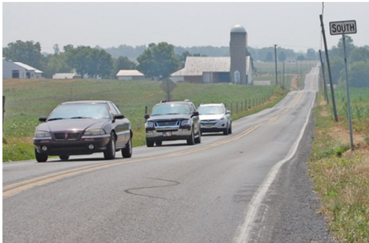
PA Route 416 south from Shimpstown Road typifies the study area's narrow pavement widths and high prevailing speeds
